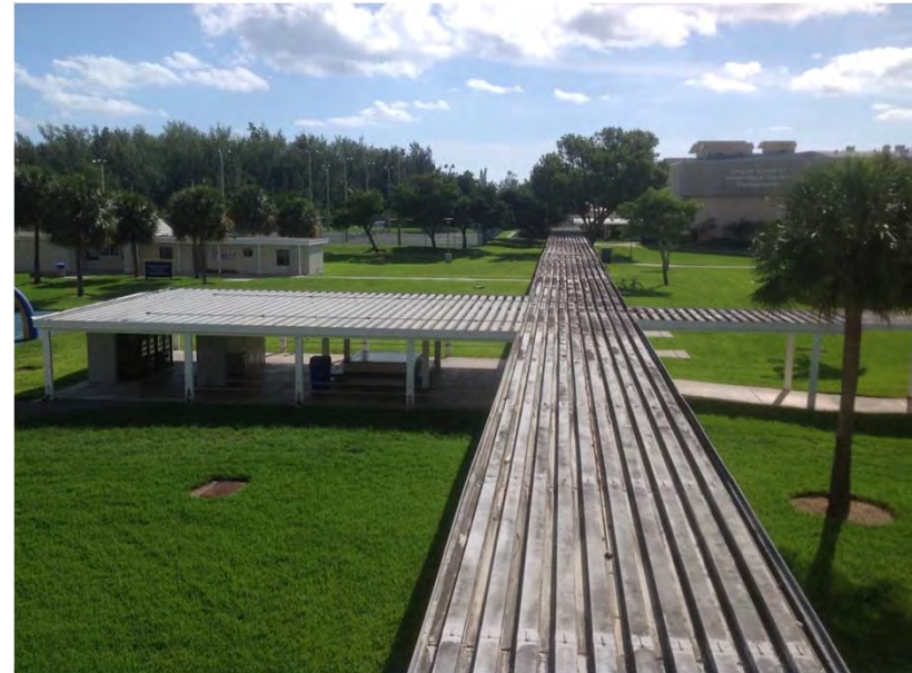
Repair of existing covered walkways
