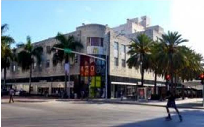
New facilities in the community
