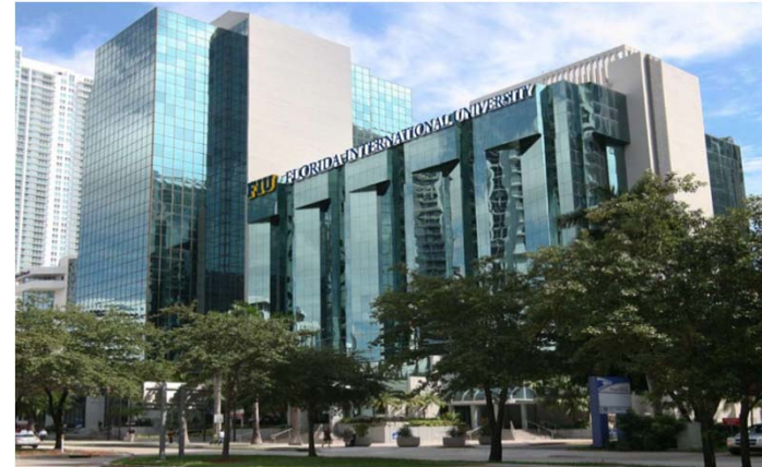
New facilities in the community
