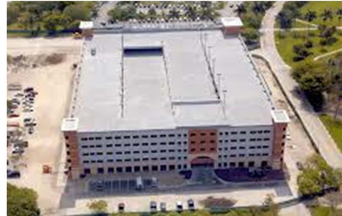
Need for additional parking structures
