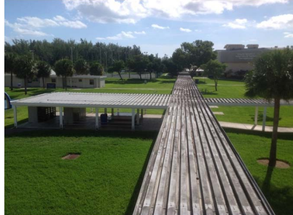
Need repairs to existing BBC covered walkways
