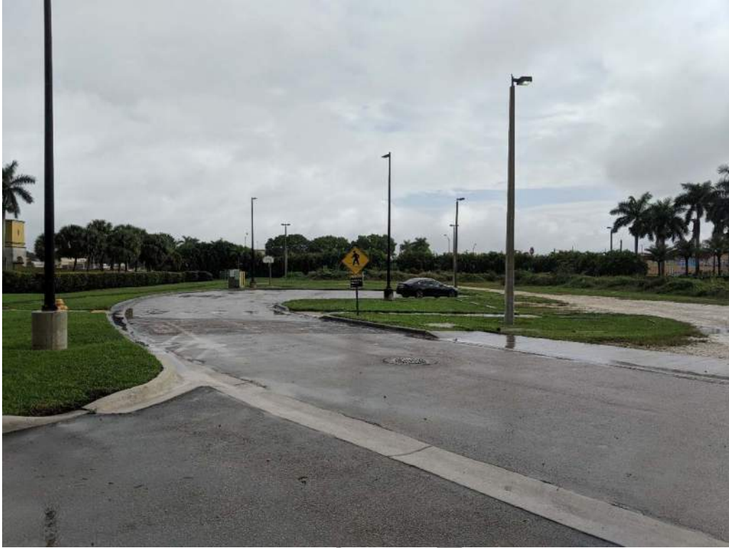
Photo 5: Western portion of the property, facing east.
