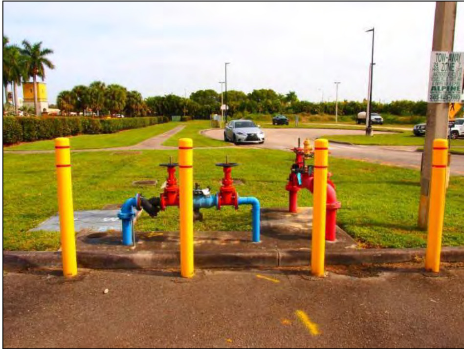
Figure 16: Utilities along the Western Boundary of the Archaeological APE, Facing East
