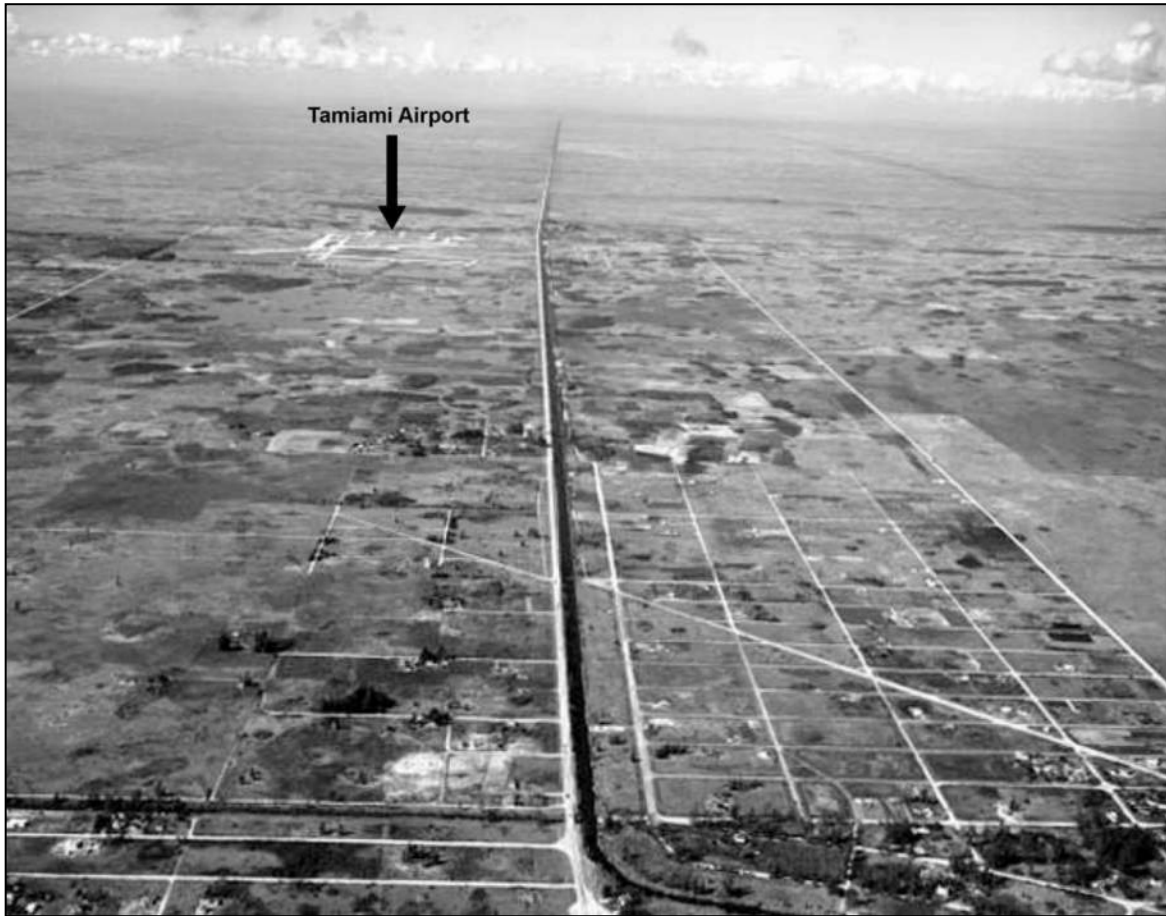
Figure 9: 1947 aerial photograph showing Tamiami Trail (US 41) looking west with Tamiami Airport in the left background (Courtesy of George W. Young)
